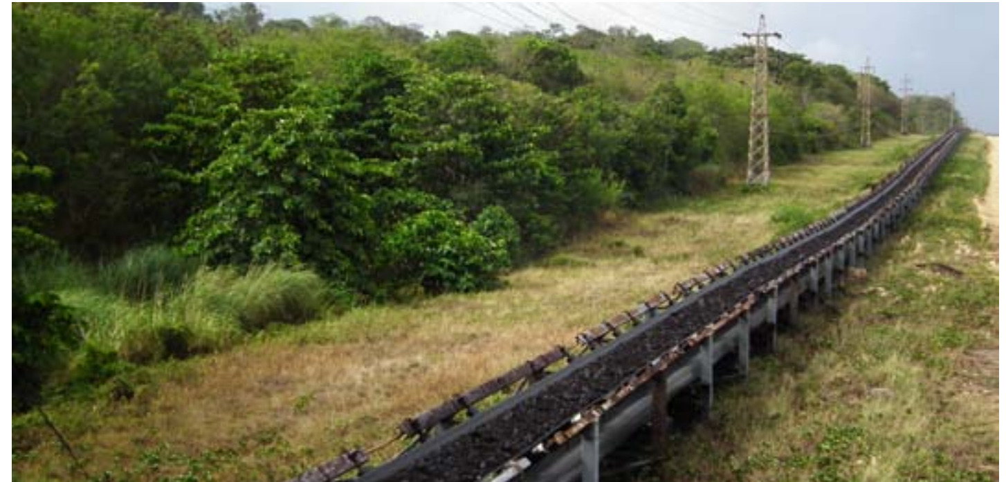
Transporting coal through conveyor for shipment to customer’s power generation needs.
